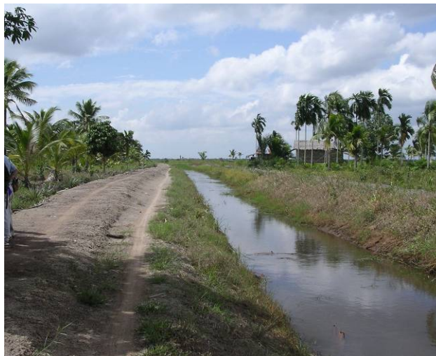
Figure 3.2 – Canal embankment shaped into farm road for motorcycles and small carts.
