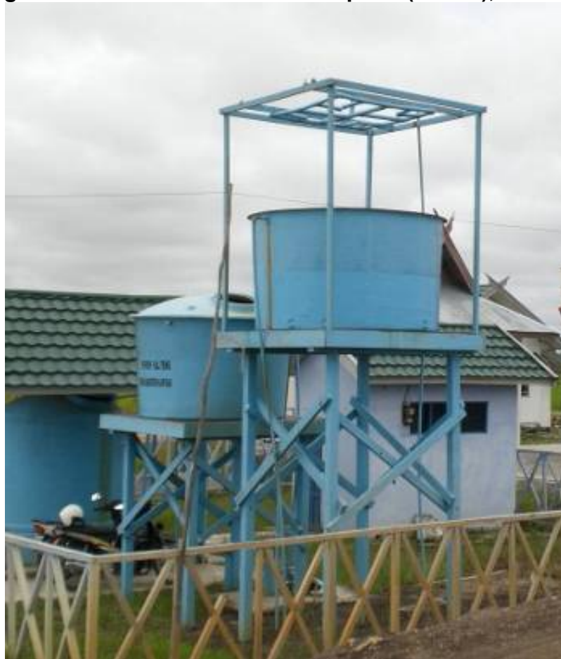
Figure 4.2 – Communal treatment plant (SIPAS), Lamunti
