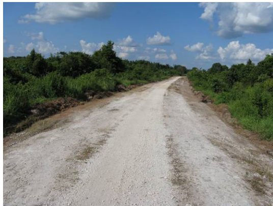
Properly constructed, with sufficiently wide shoulders
