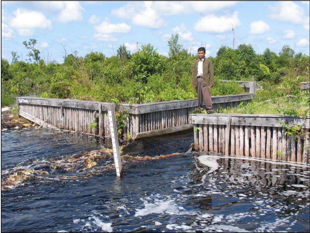
Photo 1: Dam constructed by WWF near the Sebangau NP Fire Station.
