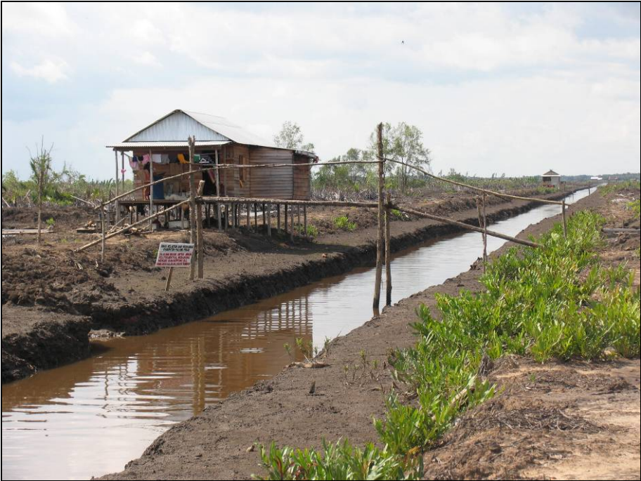
Photo 2: 600 ha of semi-intensive ponds are under construction.
