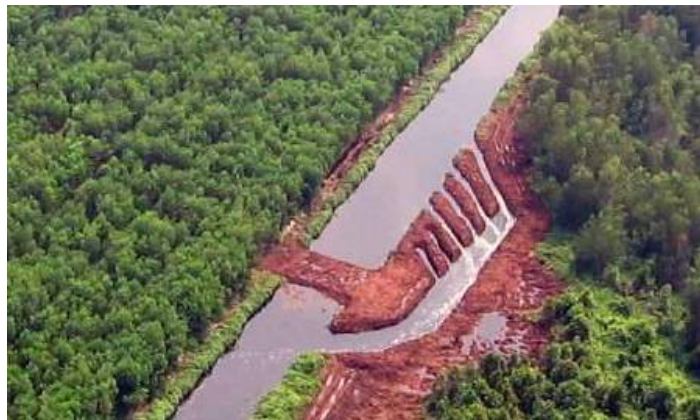
Figure 4.4 – Kampar, Sumatra, peat dam with narrow bypass
