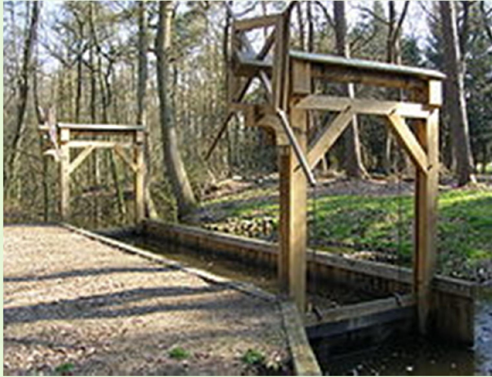
Model of early river pound lock, constructed in Lankheet water park, Netherlands
