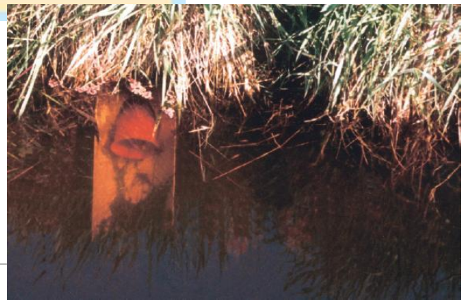
Example of tube drainage below surface water for water infiltration to groundwater.
