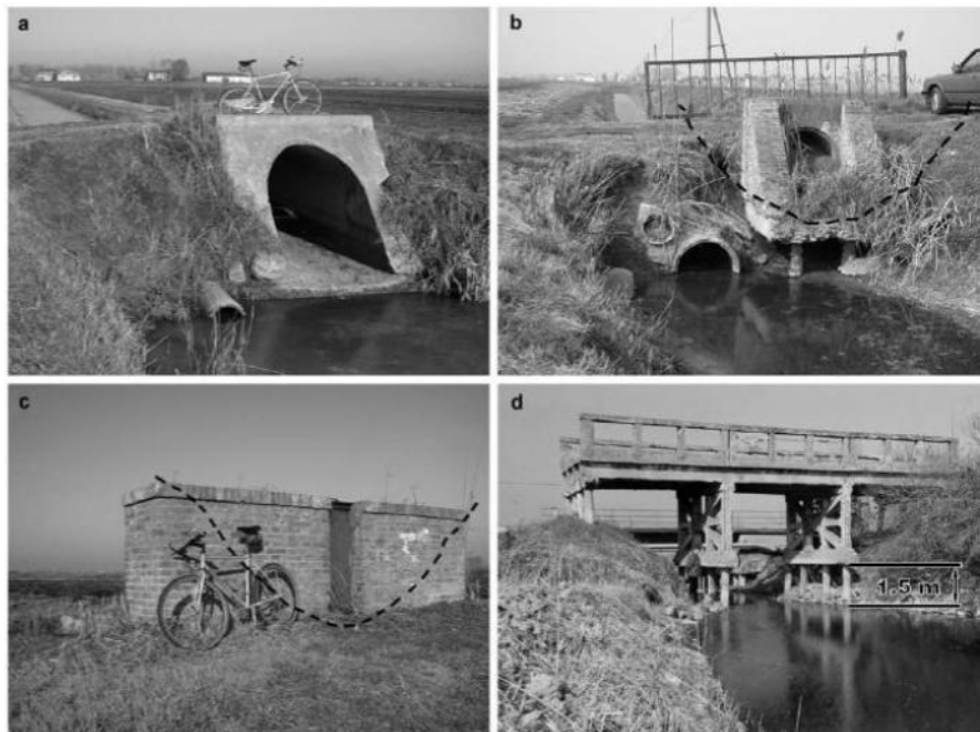
Figure 23.4. Evidence of the anthropogenic land subsidence in the reclaimed area. (a) A bridge has been turned into a useless structure: the left drainpipe helps convey the water of the channel originally flowing through the protruding infrastructure. (b) An old masonry culvert presently above the water level and substituted by two lower concrete drainpipes, the higher of which already unusable. The approximate position of the ditch section in the original configuration is sketched. (c) The protrusion of a sluice wall above the bed of an old disappeared channel. (d) An old bridge hanging over the canal bank that settled by 1.5 m.
