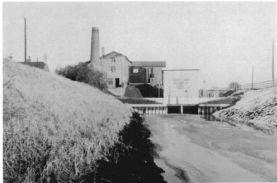
PLATE 3. The various Whittlesey Mere Pumping Stations. Photograph taken Feb. 1963 from the Engine Drain, looking E. The twin buildings to the left, adjoining the chimney, housed the original and the second pumping plants; the central building housed the 1924 diesel plant; the latest station is lower down to the right.
