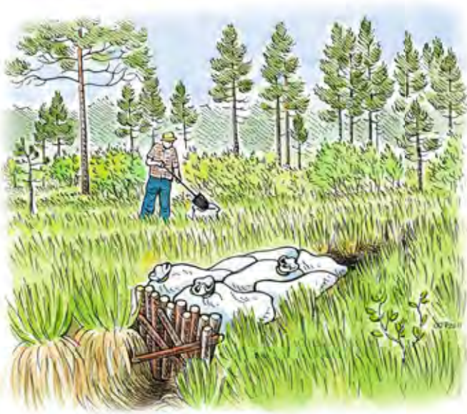
Figure 38. Jute sacks filled with compressed peat can be put in place manually to dam ditches with sensitive springs or seepage areas, for instance. Such sack dams are also suitable for use when repairing dams in restored sites where excavators can no longer work. Sacks can be fixed in place using wooden stakes hammered into the peat.
