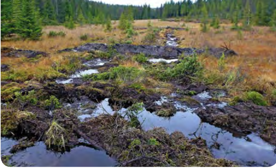
Figure 32. In wet sloping peatlands peat embankments are particularly important, since they help water to spread over the peatland rather than continuing to flow along the courses of infilled ditches. PHOTO: ULLA AHOLA.
