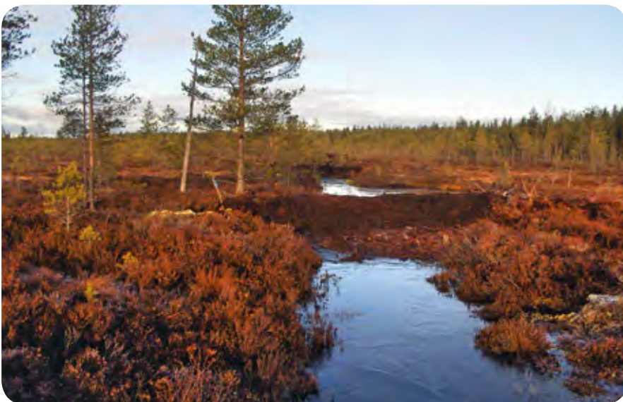
Figure 33. It may be worth making very long peat embankments in key locations with regard to water flows. In this site embankments were about 60 metres long. The dimensions of the embankments were clearly marked in the field with ribbons to ensure that the excavator driver made them long enough. This photograph was taken from the site of the infilled ditch, where water earlier flowed from right to left. The embankment was made perpendicular to the ditch line. A channel formed where peat was dug up to make the embankment, and water now flows along this channel to feed areas of flark fen which had not been drained but had nevertheless dried out. PHOTO: REIJO HOKKANEN.
