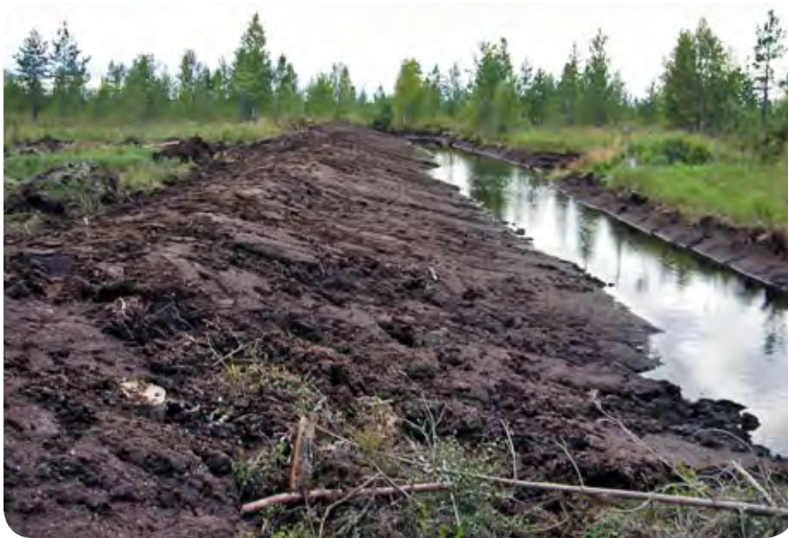
Figure 65. This peat embankment was constructed a couple of weeks before the photograph was taken. The pools excavated alongside have not yet filled with water. PHOTO: PÄIVI VIRNES, AUGUST 2007.
