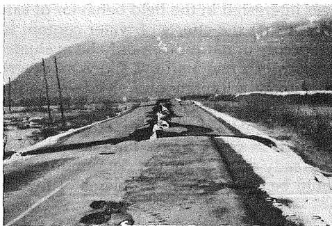
**FIG. 8.—Cracking of Embankment Associated with Lateral Spreading of Embankment in Alaska Earthquake (1984)**
