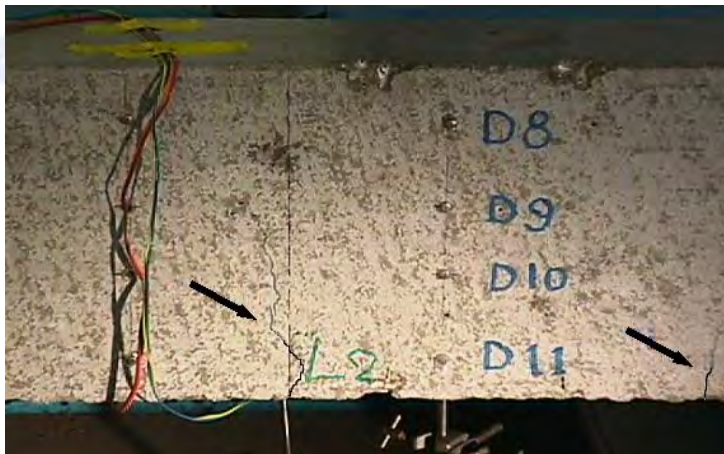
Demec Points capturing the first crack.
