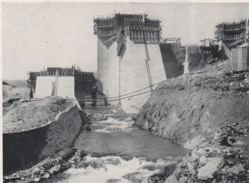
Fig. 8. Temporary openings between buttresses 8 and 9 and diversion channel
