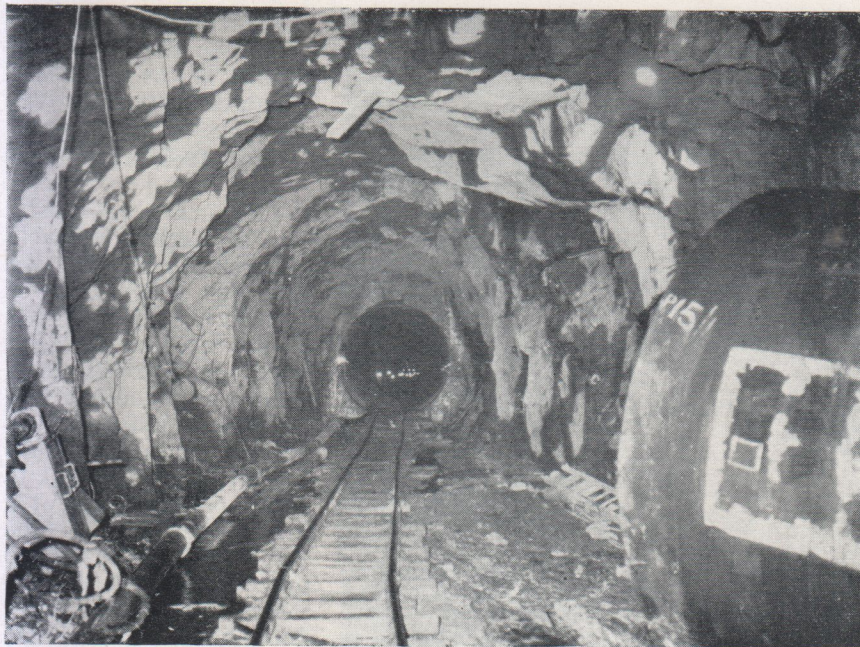
Fig. 9. View inside Nant-y-Moch to Dinas tunnel before completion of lining
