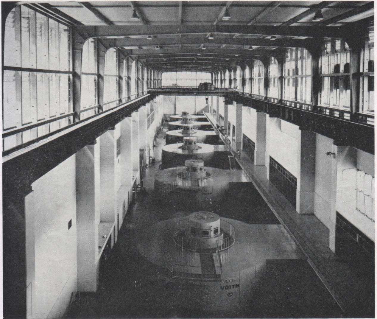
Fig. 7. Macagua No. 1 machine hall after the installation of all six machines
