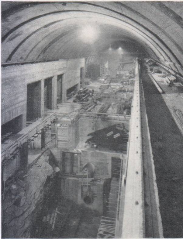
Fig. 17. Ferrera machine hall at a later stage of construction
