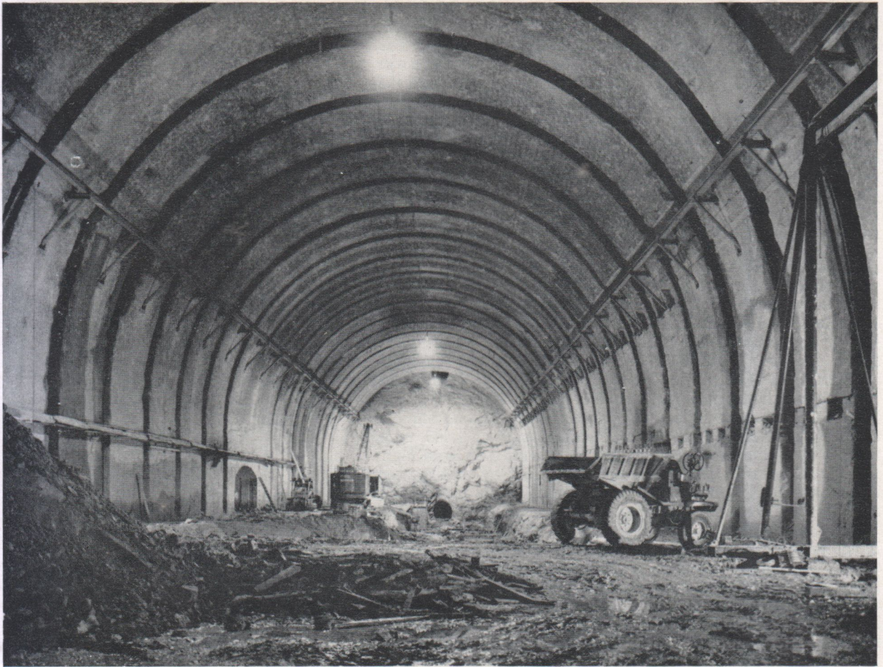
Fig. 15. Ferrera machine-hall cavern in course of excavation
