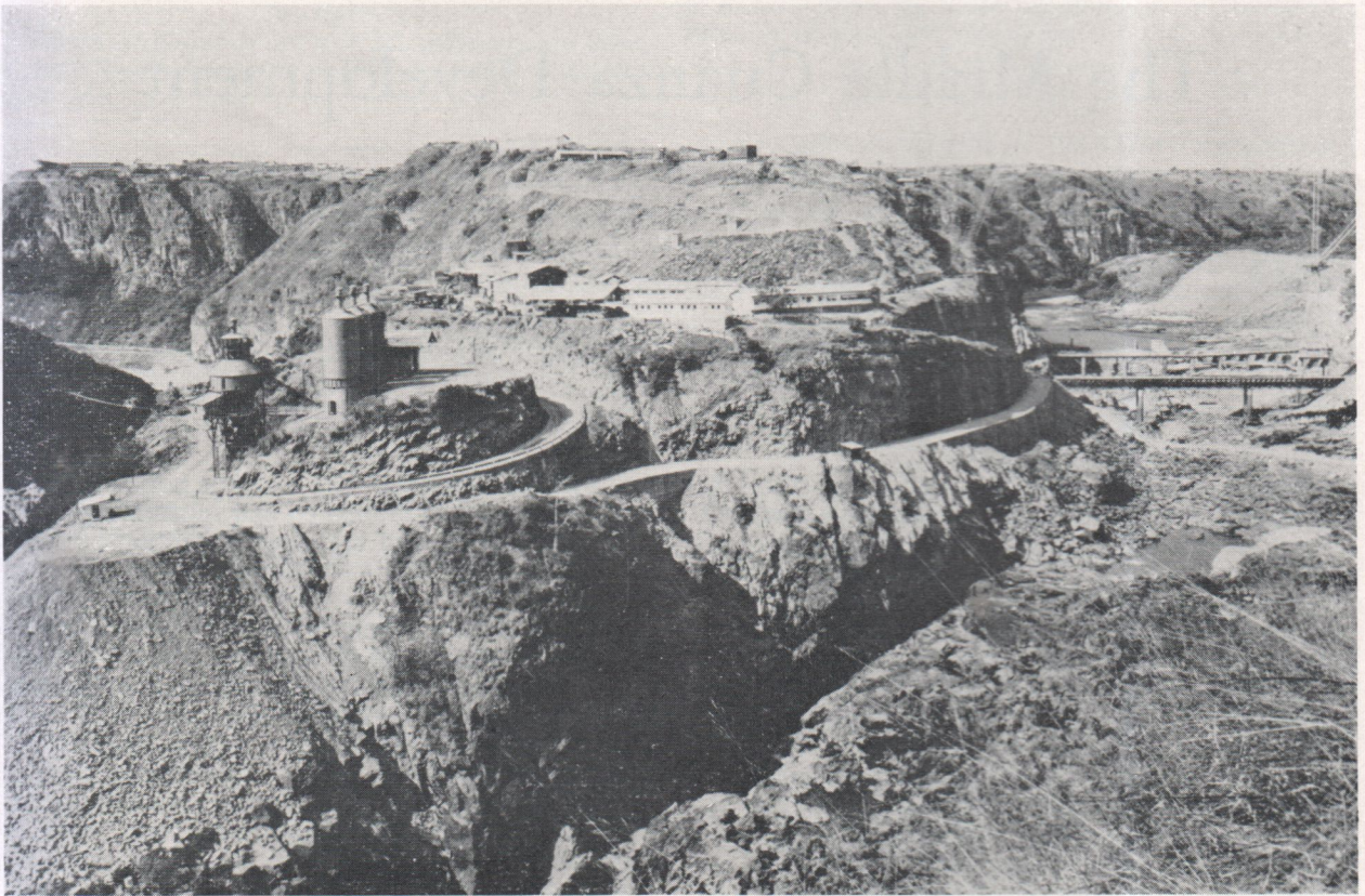
Fig. 12. In this photograph can be seen the two sides of the river bend which are connected by the underground power plant below the hill in the centre. The concrete-mixing plant is in the foreground and the dam site on the extreme right
