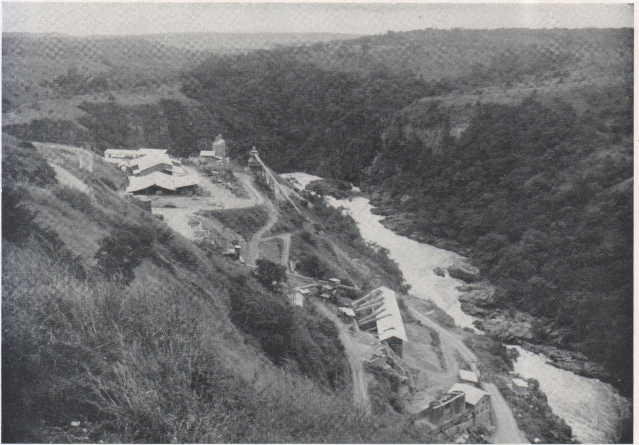
Fig. 11. A general view of the crushing, screening and washing plant
