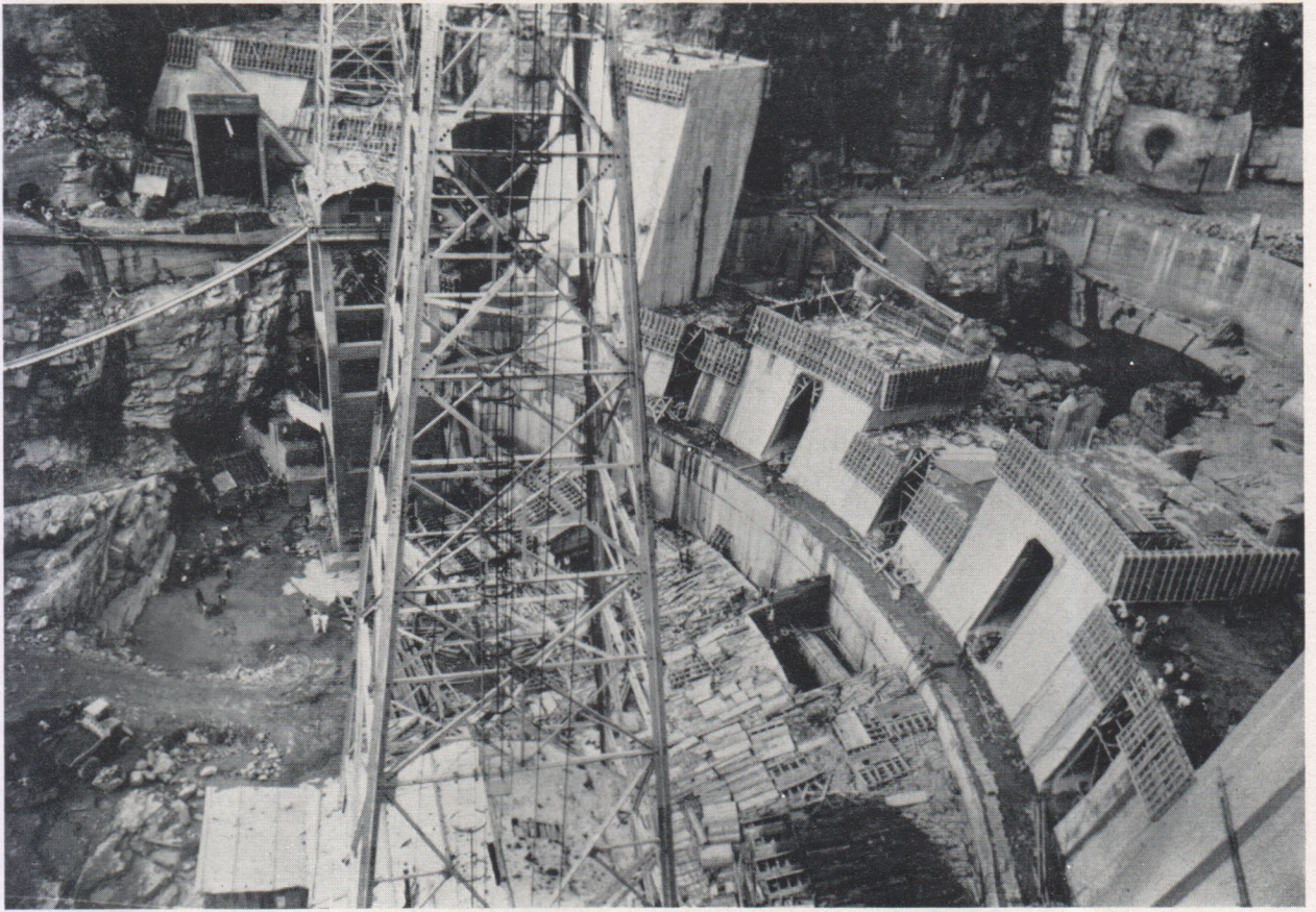
Fig. 10. A recent view of Cambambe dam under construction
