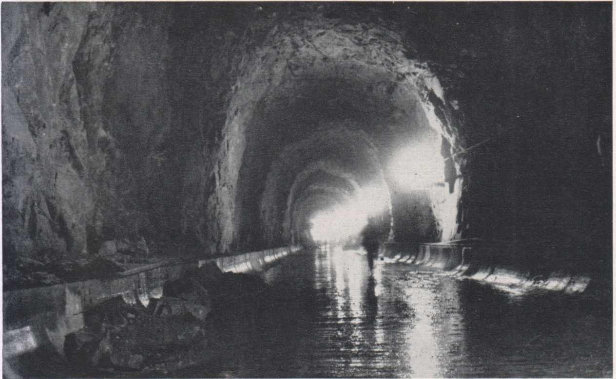
Fig. 9. A view inside the combined bottom-outlet and diversion tunnel
