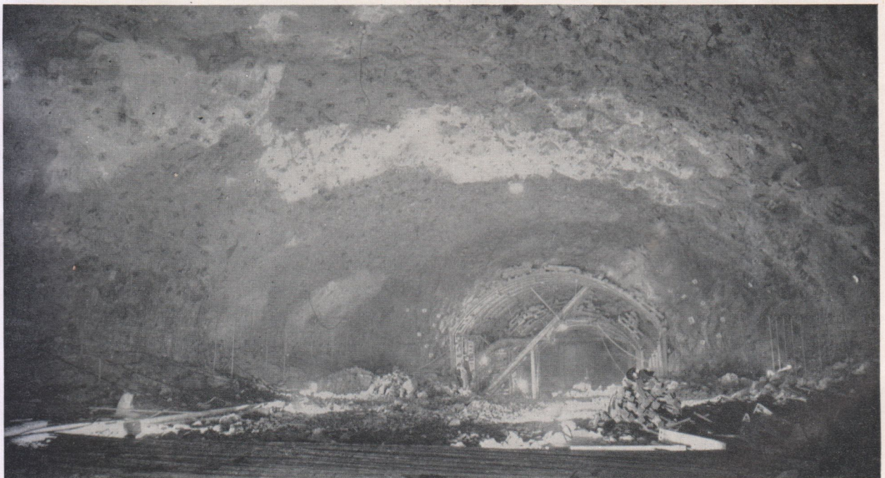
Fig. 14. Excavation for transformer hall showing complete rock bolt support
