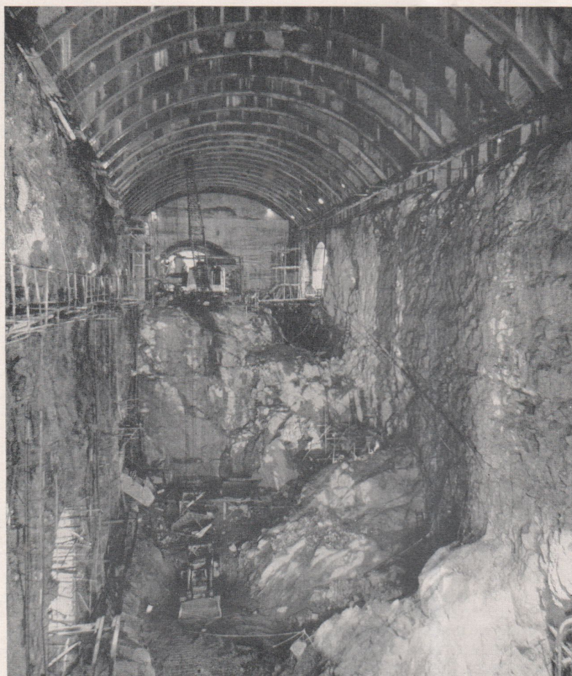
Fig. 13. Excavation for Tumut I power station
