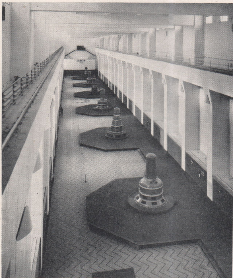
Fig. 8. Machine hall of Henri Poincaré station
