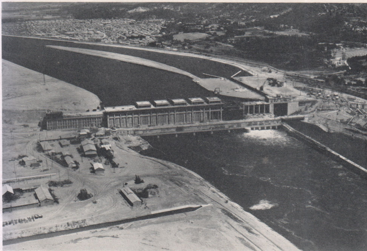
Fig. 3. Upstream view of Donzère power station showing canal lock and tailrace
