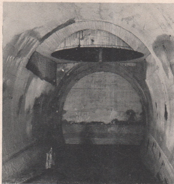
Fig. 12. Discharge tunnel and turbine draught tube of Mullardoch subsidiary generating station
