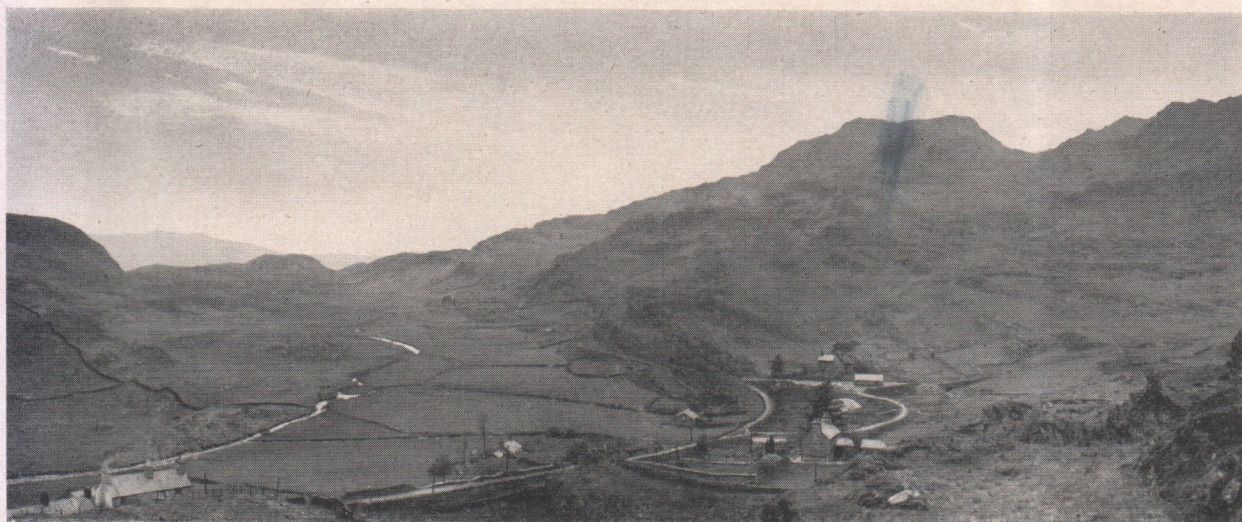
Fig. 1. Proposed site of the lower storage reservoir on the Afon Ystradau, Ffestiniog project
