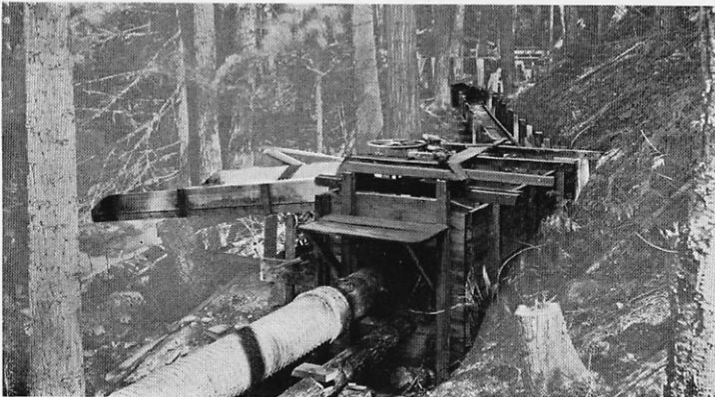
Fig. 42. Typical Flume and Pressure Box for small installation, showing headgate, pipe-intake, and spillway in place
