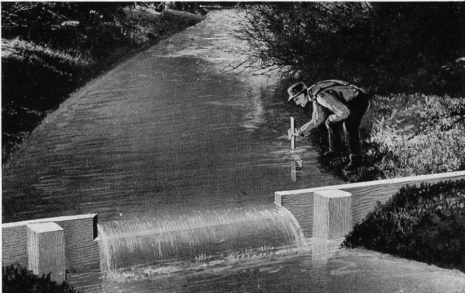
Fig. 41 A Weir correctly constructed, showing the method of measuring the amount of water flowing in a stream
